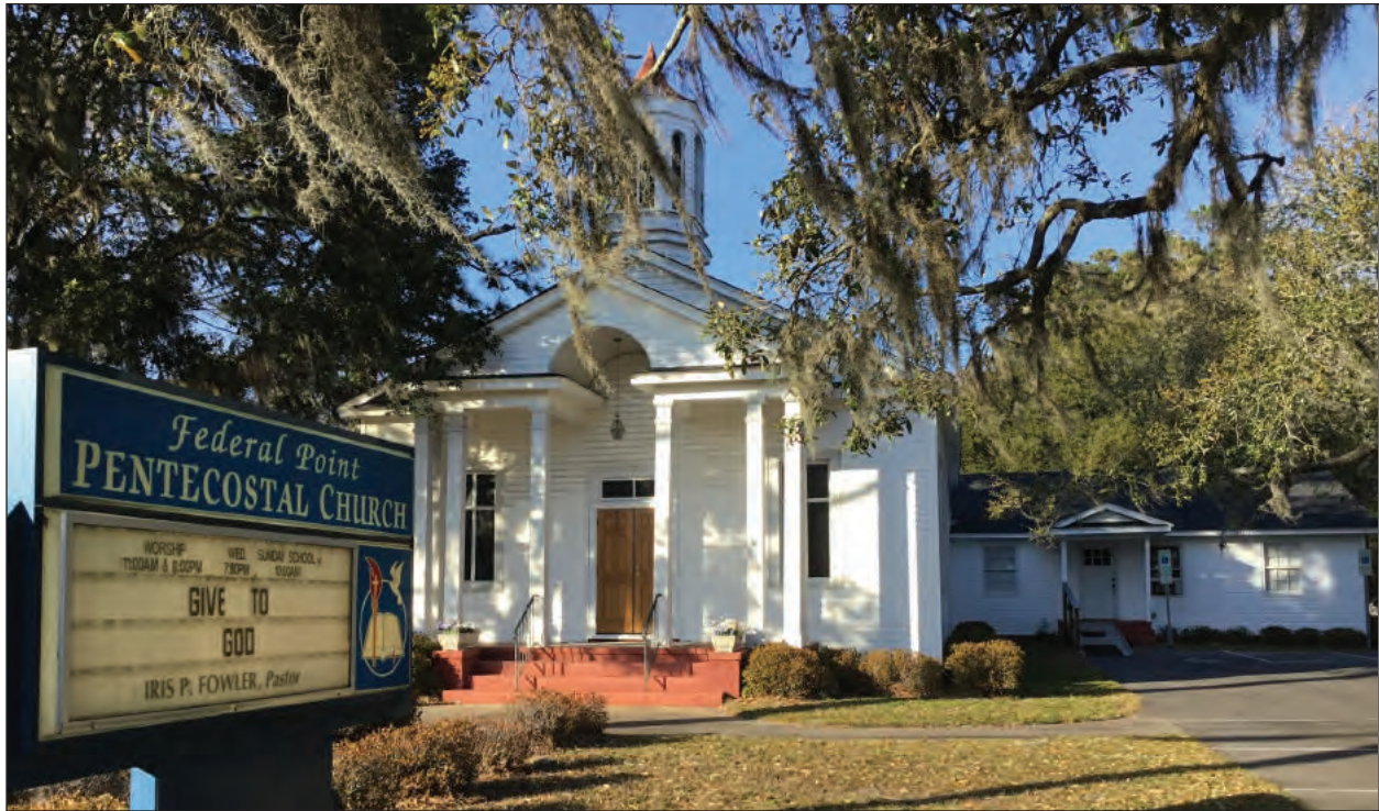
Figure 9.1. Façade, Looking South
