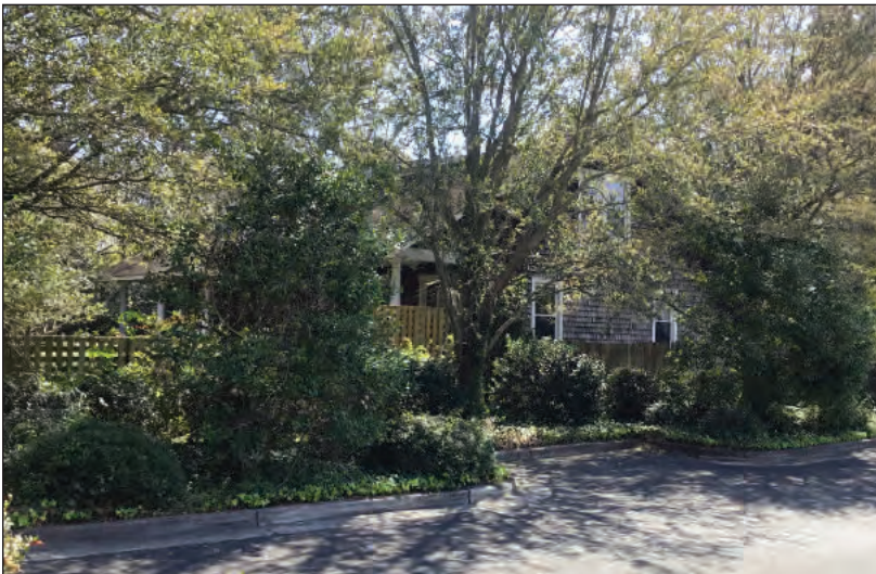
Figure 8.5. West Wall, Looking Southeast
