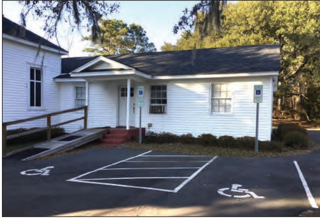
Figure 9.6. East Wing, Looking North
