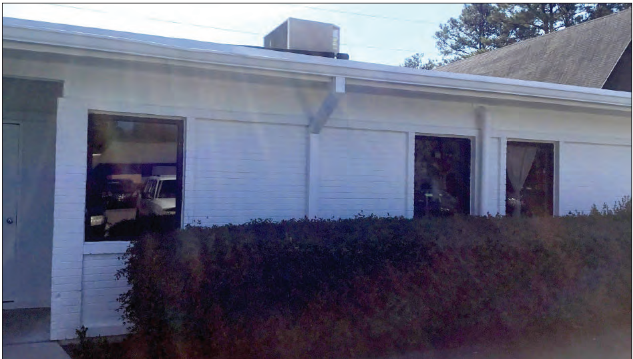
Figure 3.6. Detail of Rear Wall and Windows, Looking Southeast
