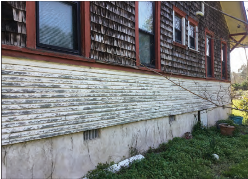
Figure 6.3. West Wall, Showing Variety of Wall Materials
