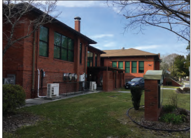
Figure 11.3. East Wall of 1914 Addition
