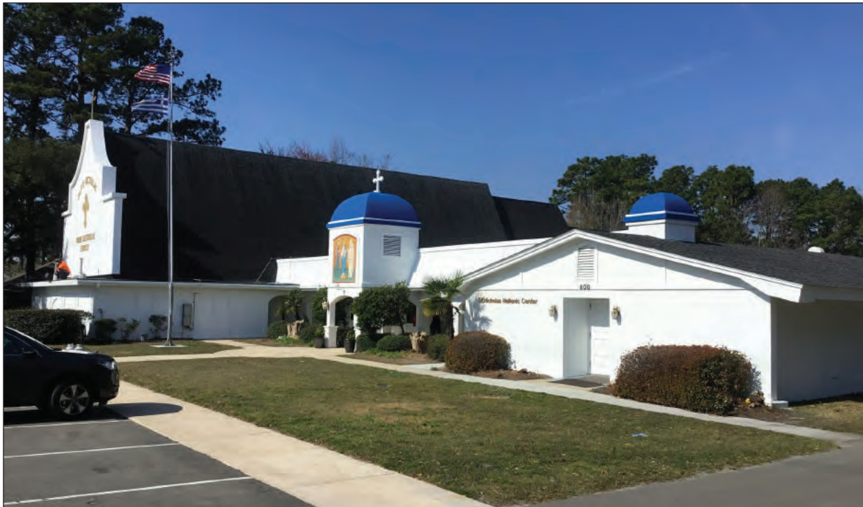
Figure 3.3. Church Façade, Looking Southwest
