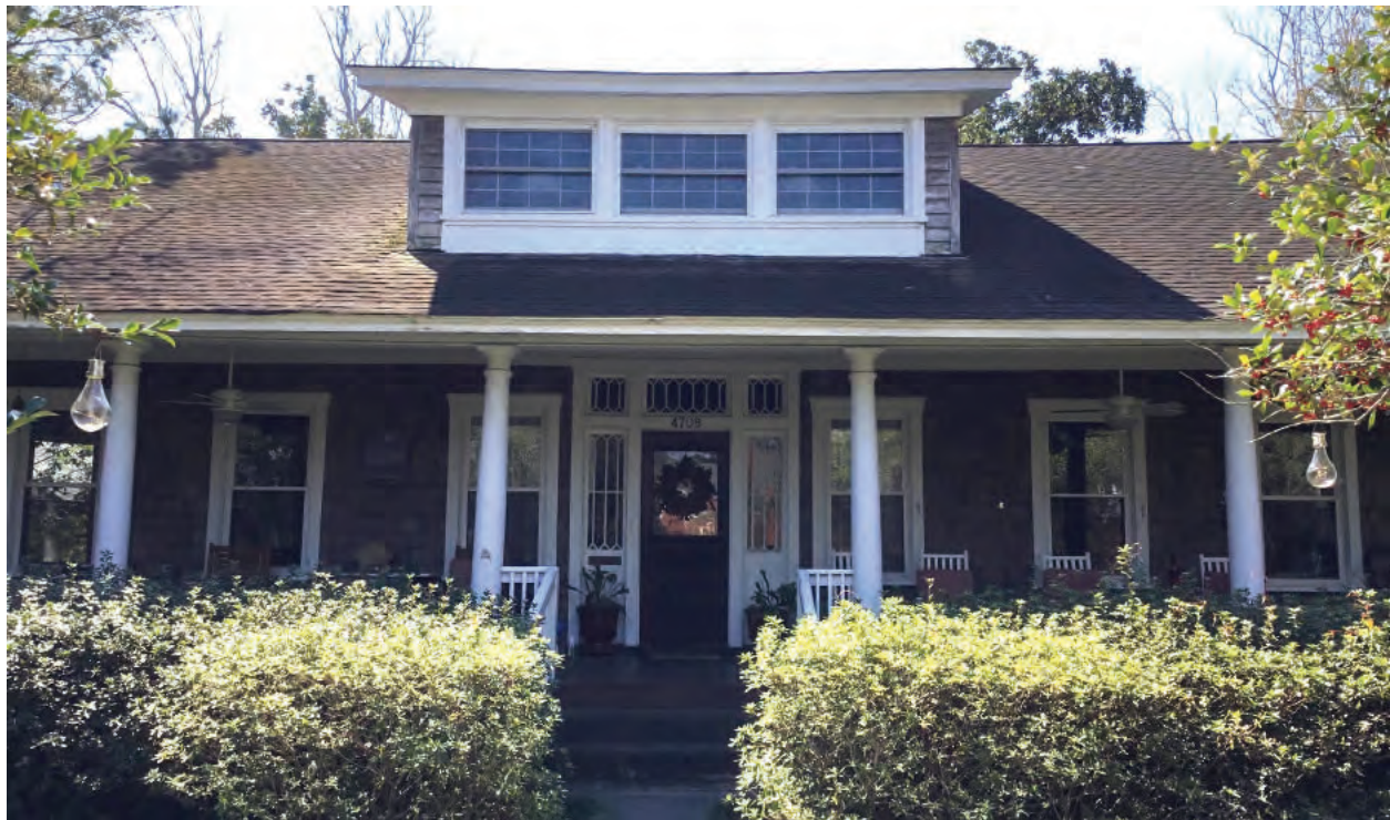
Figure 8.1. Façade, Looking South
