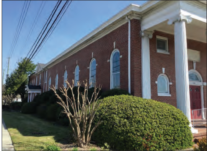
Figure 10.3. West Wall of Sanctuary and 1956 Rear Addition, Looking North
