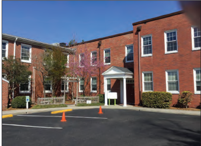
Figure 10.4. South Wall of 1956 and 1961 Additions
