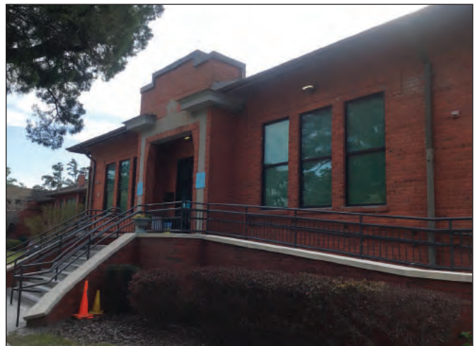
Figure 11.4. East Wall/Entrance of 1930s Addition
