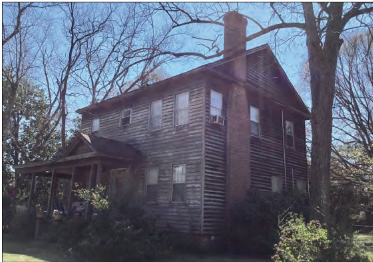
Figure 7.3. Façade, Looking South
