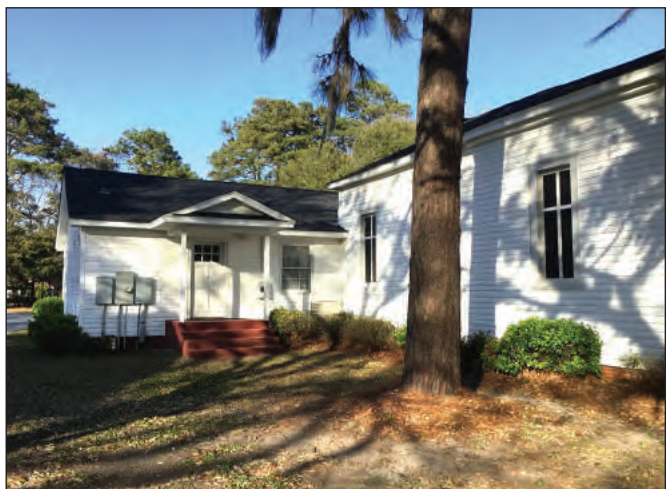
Figure 9.5. West Wing, Looking Northeast
