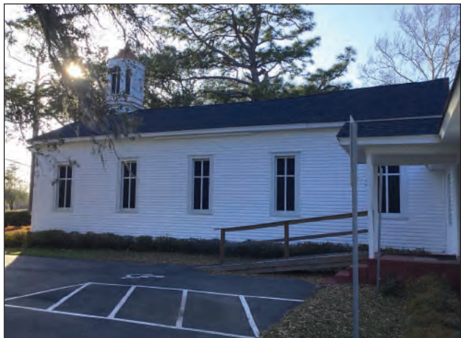
Figure 9.4. East Wall of Sanctuary, Looking West
