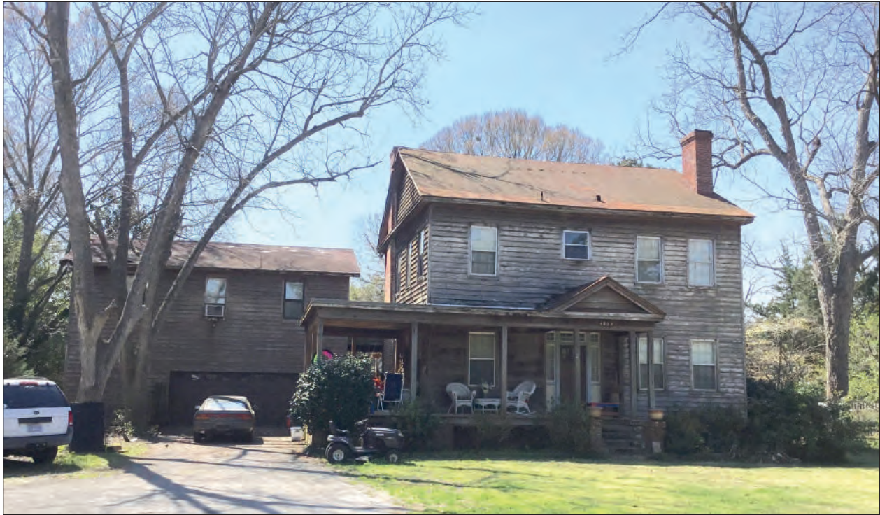
Figure 7.1. Façade, Looking South
