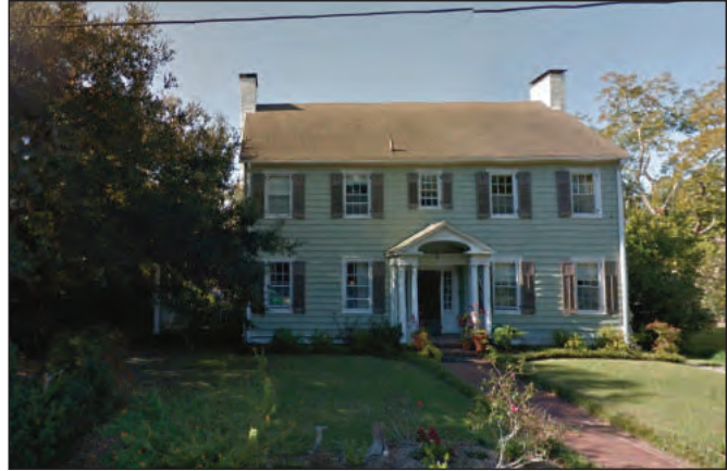
Figure 7.6. 109 N. 15th Street
