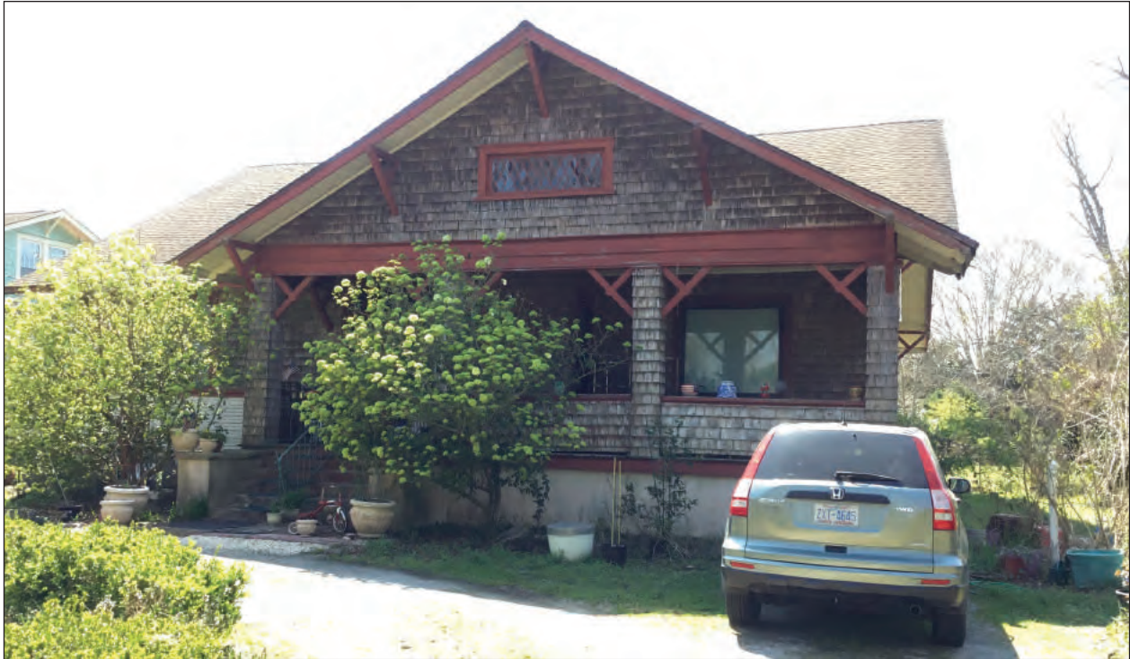
Figure 6.1. Façade, Looking South
