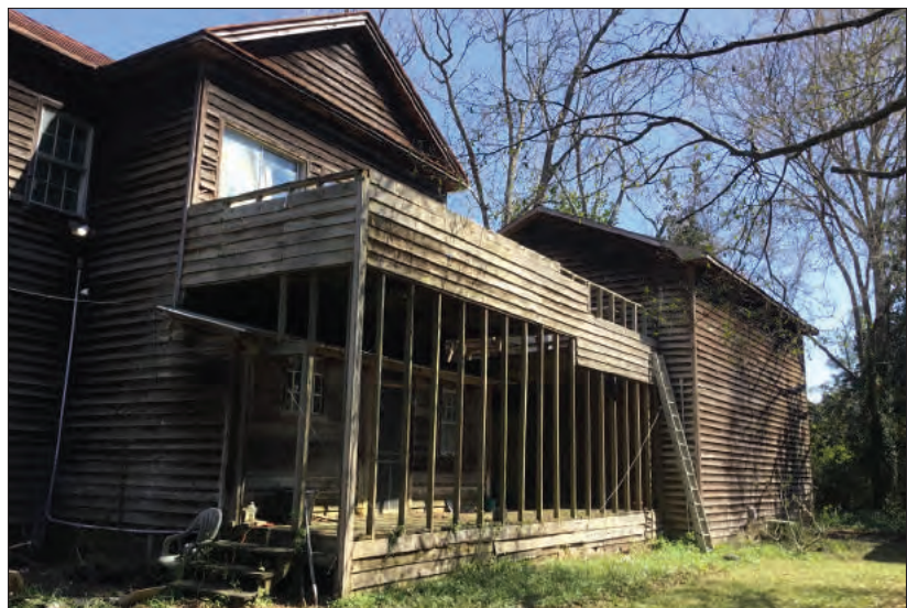
Figure 7.4. Façade, Looking South
