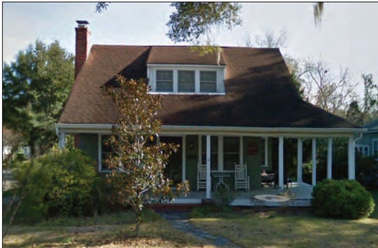
Figure 6.13. 212 N. 16th Street
