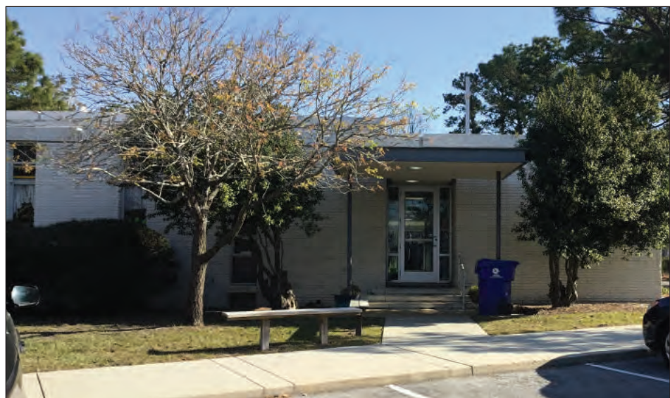
Figure 4.4. 1963 Education Building, Looking Northeast
