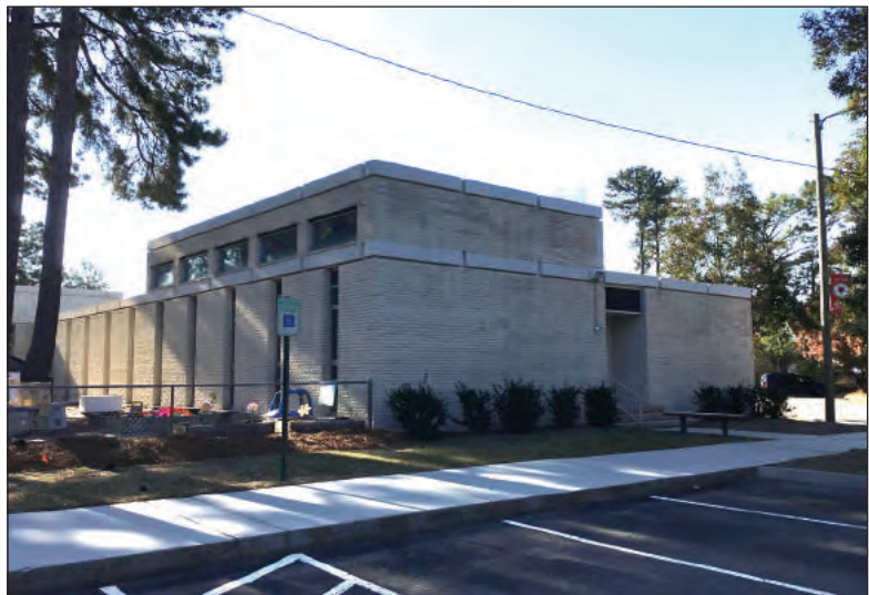
Figure 4.12. Education Building Addition
