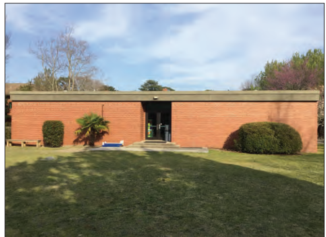
Figure 11.5. West Wall of 1956 Addition
