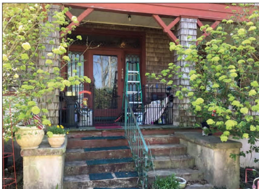
Figure 6.4. Front Entrance, Looking South
