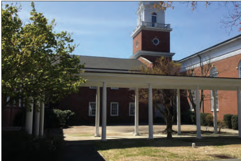
Figure 5.6. Covered Breezeway and Wing Addition, Looking Southwest
