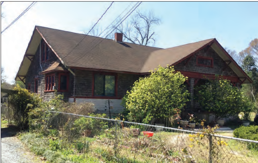
Figure 6.7. Oblique View Showing Front and East Walls
