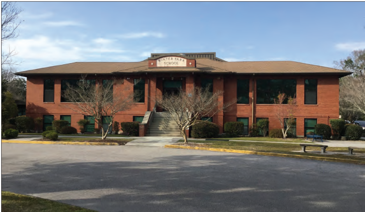
Figure 11.1. Façade of Oldest Section of Winter Park School, Looking North
